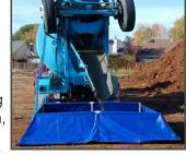
prevents runoff from entering it can be constructed. The liner should be at least 10 millimeters and leak free.
